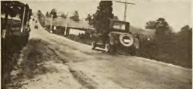
FIG. 18.—Test 20, also on an 18-foot concrete road, shows that the good shoulders permit full use of the surface, but the curve to the right just beyond the point of observation and the obstruction of the view of the right-hand traffic both cause a movement of the traffic toward the center, resulting in a center peak of traffic concentration. The presence of a center line would probably counteract this tendency
